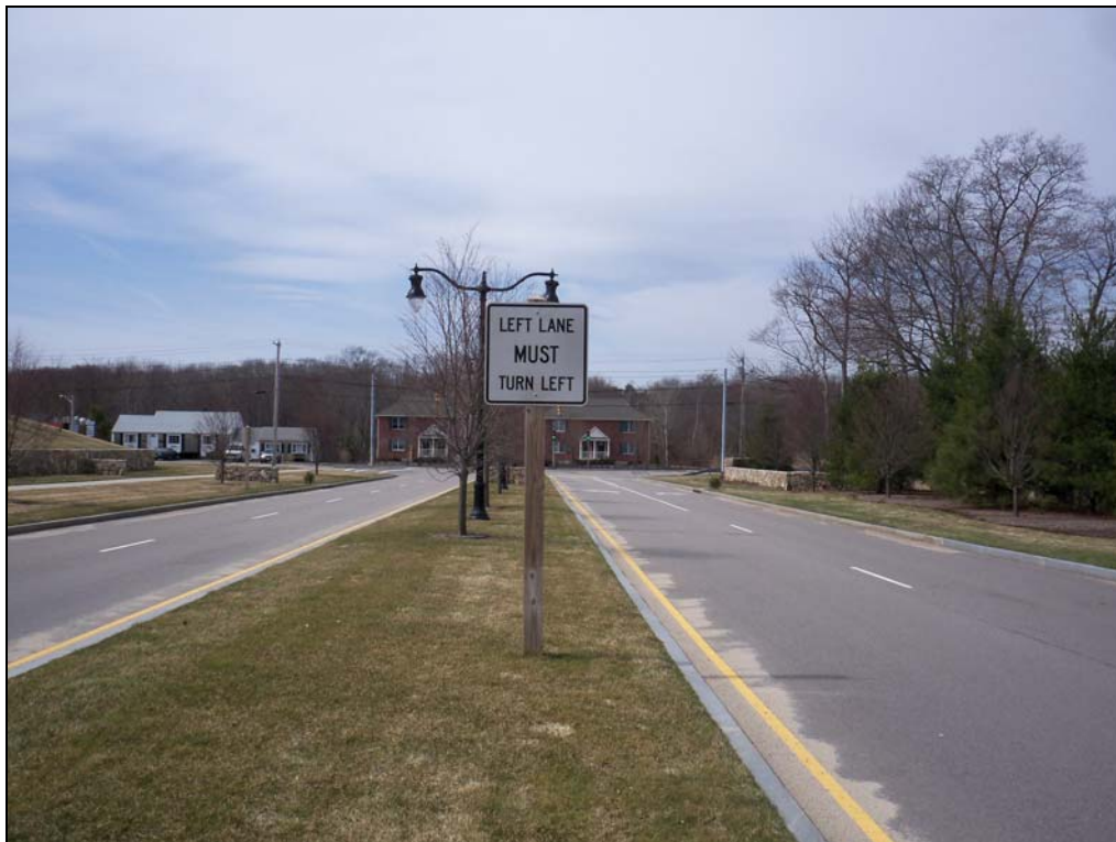
Figure A-1 Shea Drive looking west toward Route 18
