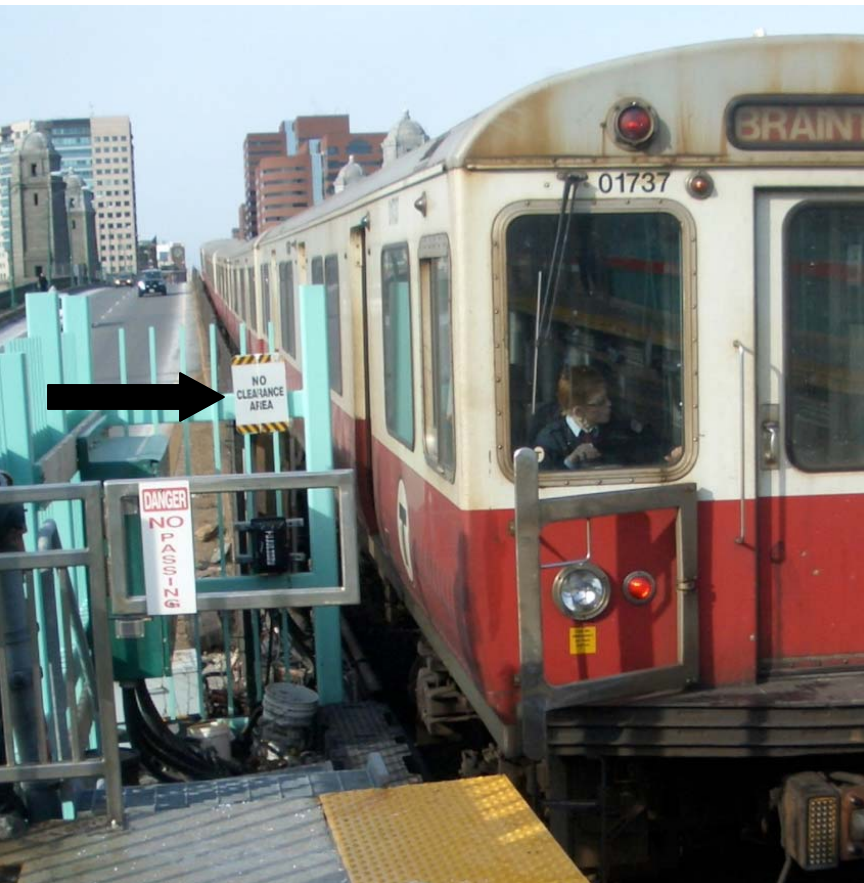
Longfellow Bridge (does not meet MBTA standards)
