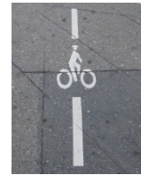
Bike loop detector pavement marking
