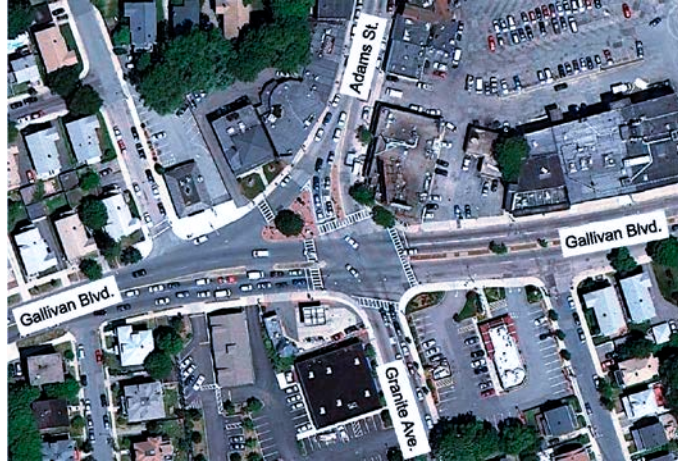
Gallivan Boulevard at Granite Avenue/Adams Street
