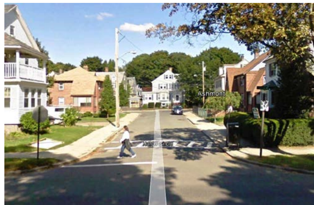
Gallivan Boulevard at Huron Circle: Curb ramps and crosswalk are not aligned to allow pedestrians to stay within the bounds of the sidewalk and the pedestrian desire line.
