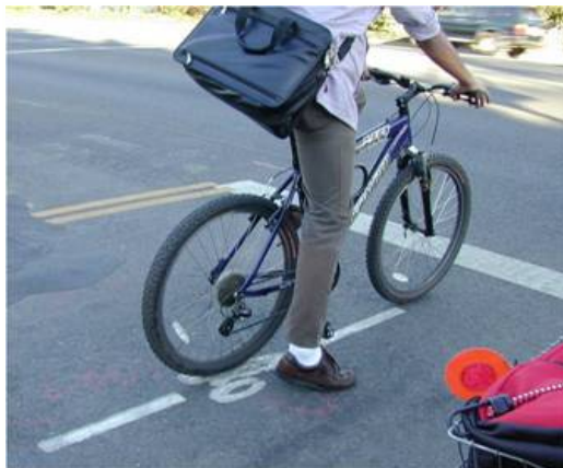
Bicycle detector pavement marking
