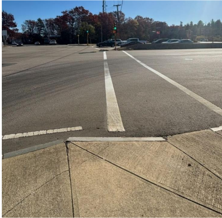
Figure 6 Crosswalk and Curb Ramp at the US Route 1 Intersection
