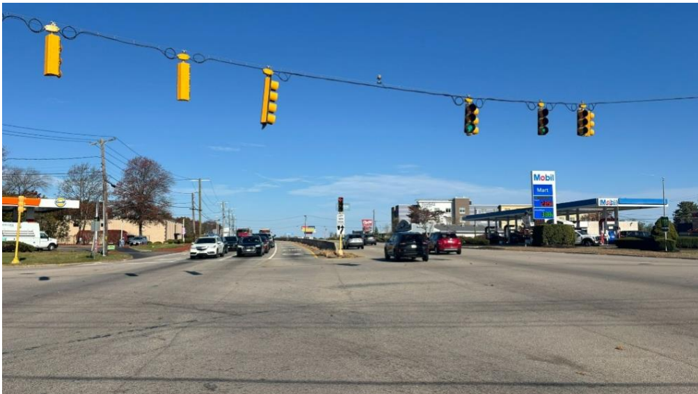
Figure 7 Lack of Turn Markings at the US Route 1 Intersection
