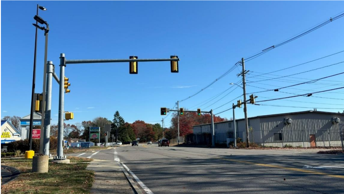
Figure 3 Signal at Walmart Entrance and High Plain Street Intersection
