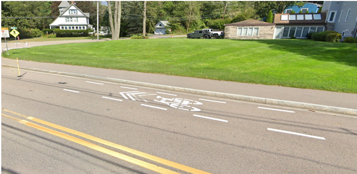
Figure 4 Shared Lane Markings South of Intersection
